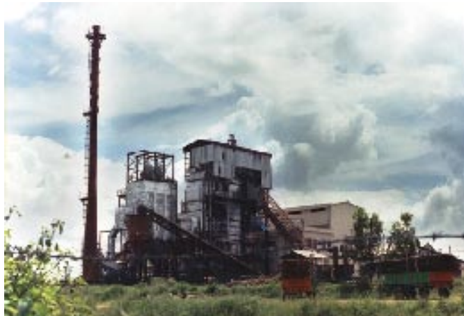
Malavalli Power Plant
